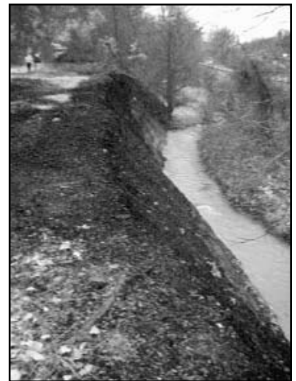
Representatives from ODNR examine a large gob pile along the banks of the West Branch Headwaters. Under the current project this area will be reclaimed.
